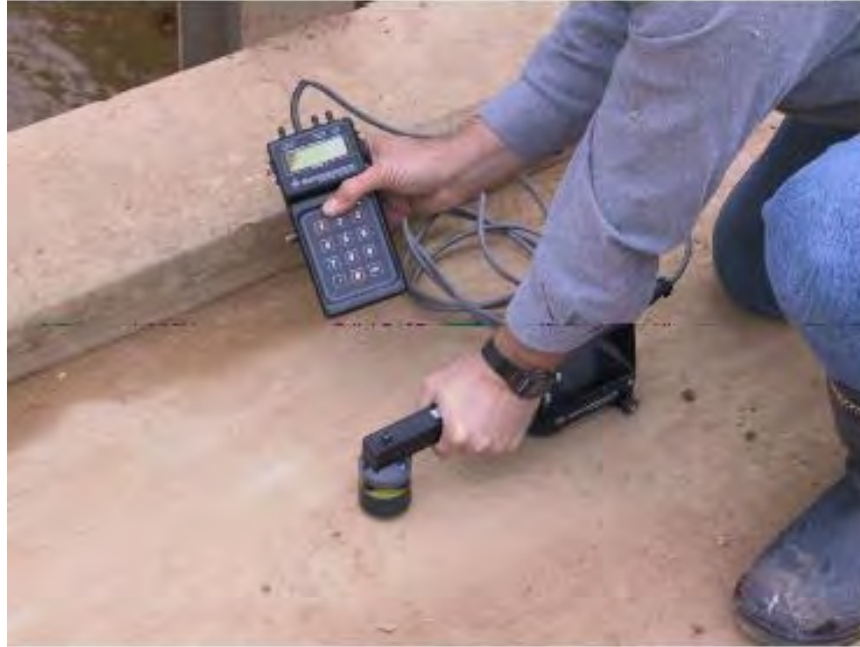
Fig. 6 SASW investigation on concrete bridge deck with hand-held IE/SASW gauge
