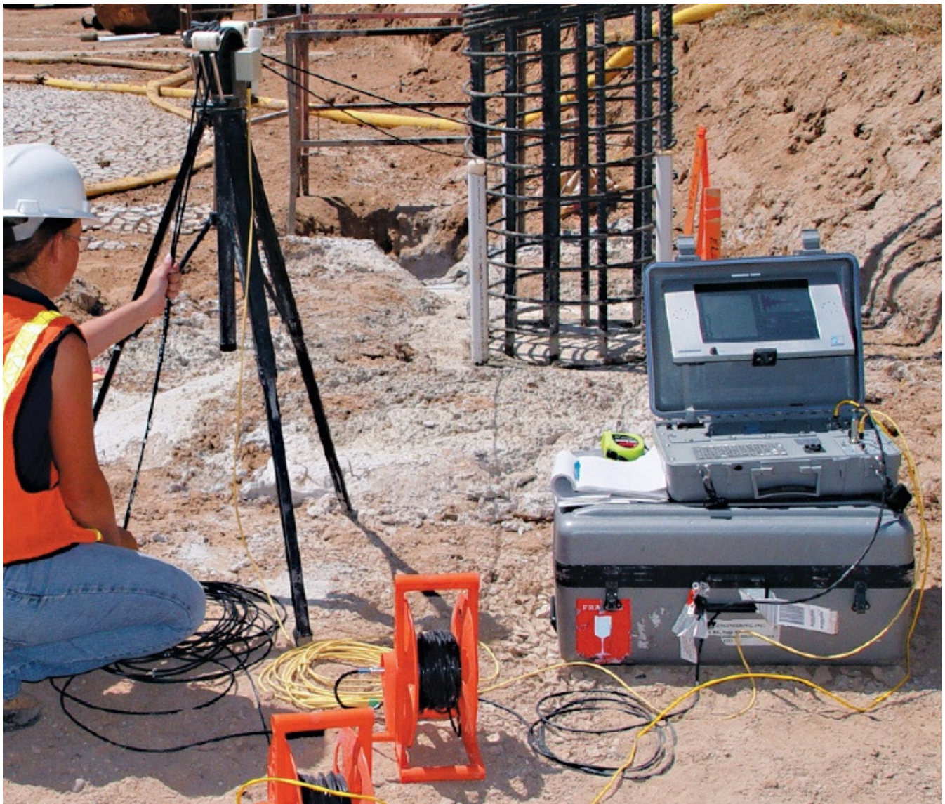
Photo showing field testing setup and procedure
