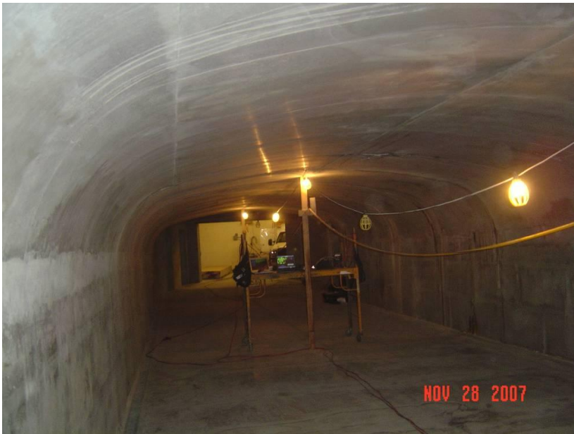
Figure 4 - Longitudinal view of the cast-in-place pedestrian tunnel
