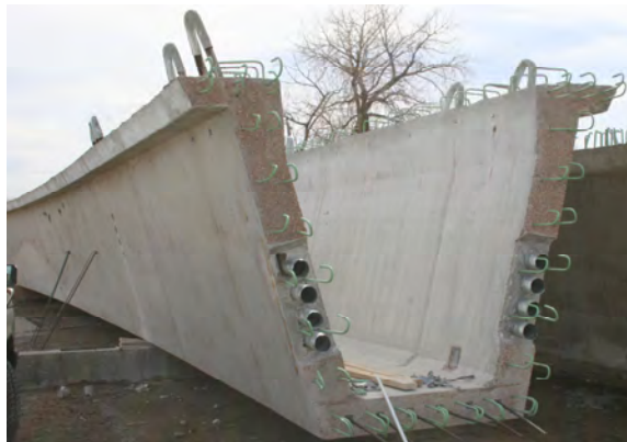
Figure 2 – U-Shaped Bridge Girder with Eight Empty Ducts - West End View
