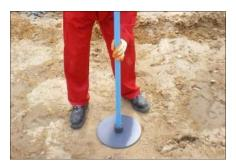
2. As filling continues, additional tube is added and care must be taken to ensure that the access tube is not damaged and that it remains vertical. When the fill reaches the elevation of the next Target, the area around the access tube must be made level and compacted.
