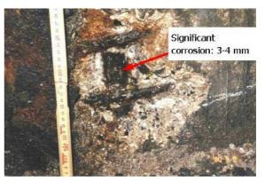
Example of exposed corroding reinforcement
